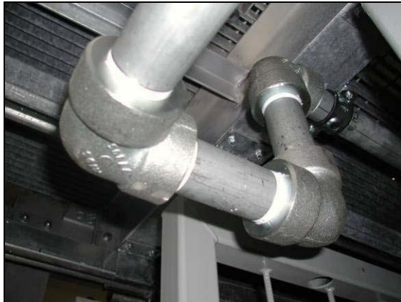
Figure 4.2 Piping system fittings
