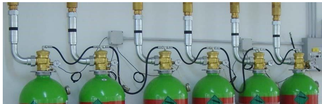
Figure 3.22 Pilot pneumatic connection
