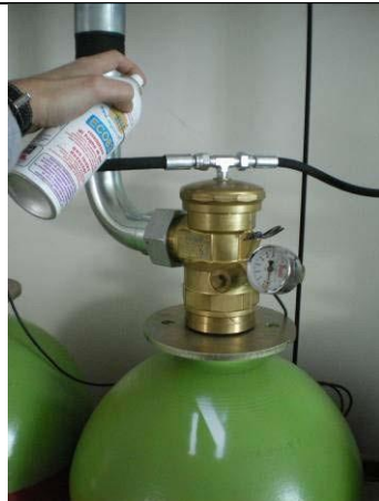
Figure 5.3 Pneumatic circuit test, step 4
