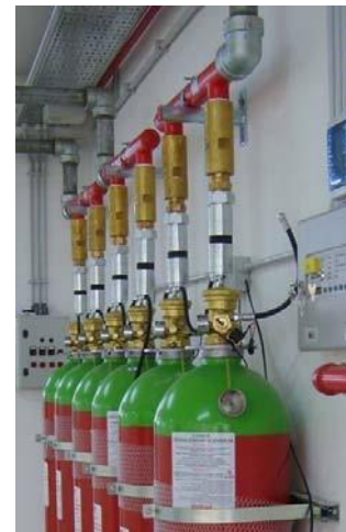
Figure 3.10 Manifold installation
