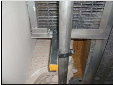
Figure 4.1 Piping system supports
